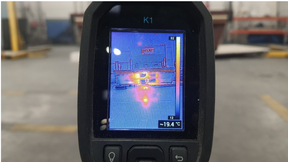
Figure 49: Thermal Camera View to Check for Smouldering of Elements
