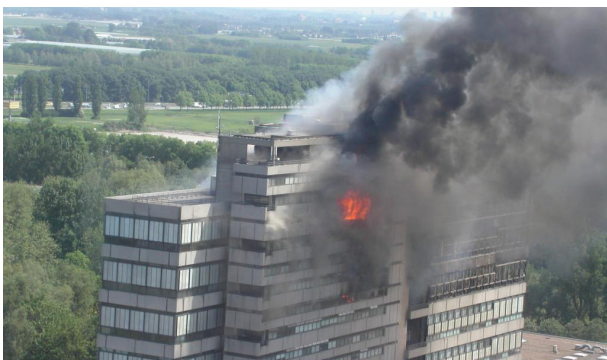
Figure 2: TU Delft department of Building and Architecture on fire: building completely demolished by a travelling compartment fire
