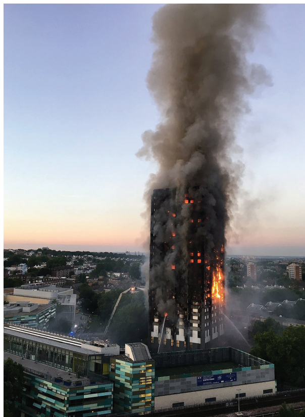
Figure 1: Grenfell tower fire, London
