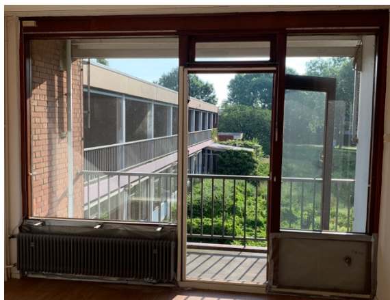
Figure 3 Non-load-bearing façade with the parapet closed panel
